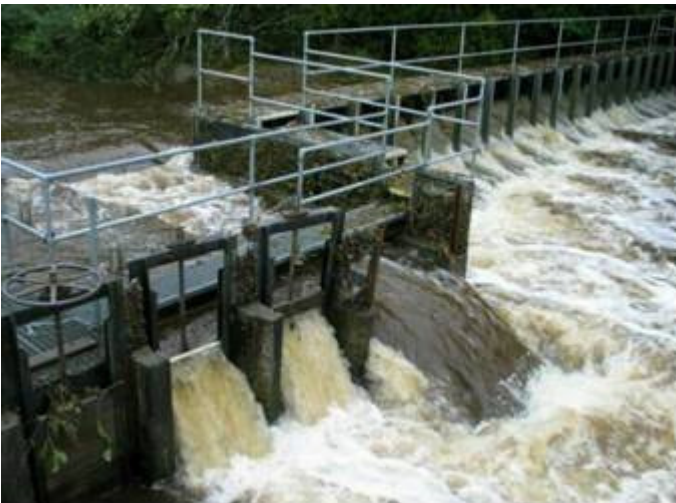
Figure 11 -- Failure of weir to restrict passage during a period of high flows on Minter Creek, WA.
