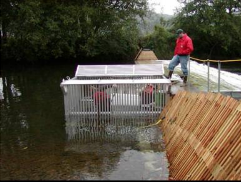
Figure 10 -- The Gray's River, WA weir, a resistance board/fixed panel design utilizing fixed wooden panels. Credit R. Walton.
